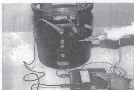
Measuring the Field Coil Insulation Resistance
